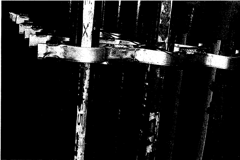
Figure 2 – Photo showing UNS S35315 anti-vibration straps used in an auxiliary steam boiler. This unit was installed at a natural gas fired co-generation plant. UNS S35315 replaced UNS S30815 and UNS N08330 as the material of choice. UNS S35315 has been used for over 4 years by this boiler OEM.
